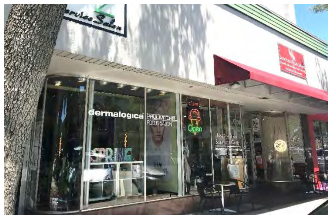
902 E New Haven Ave
