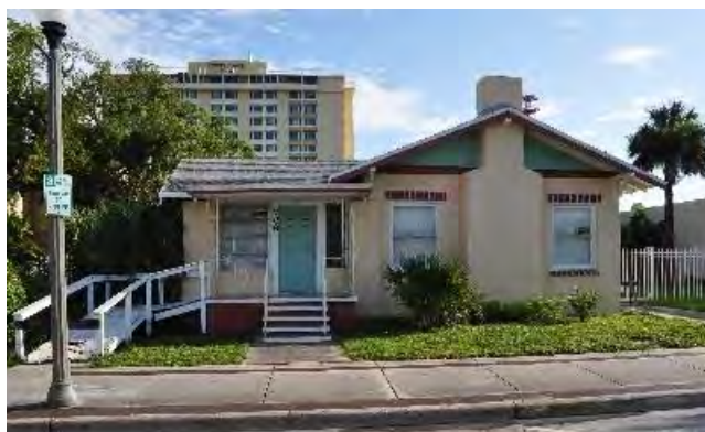
708 E New Haven Ave
