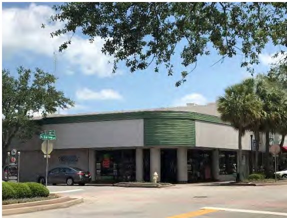
900 E New Haven Ave
