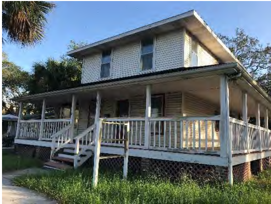
541 E New Haven Ave
