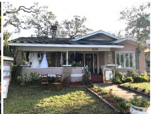
529 E New Haven Ave
