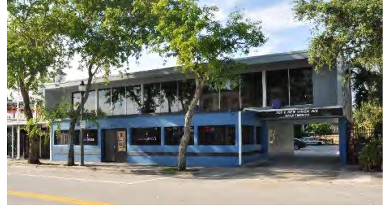
701 E New Haven Ave
