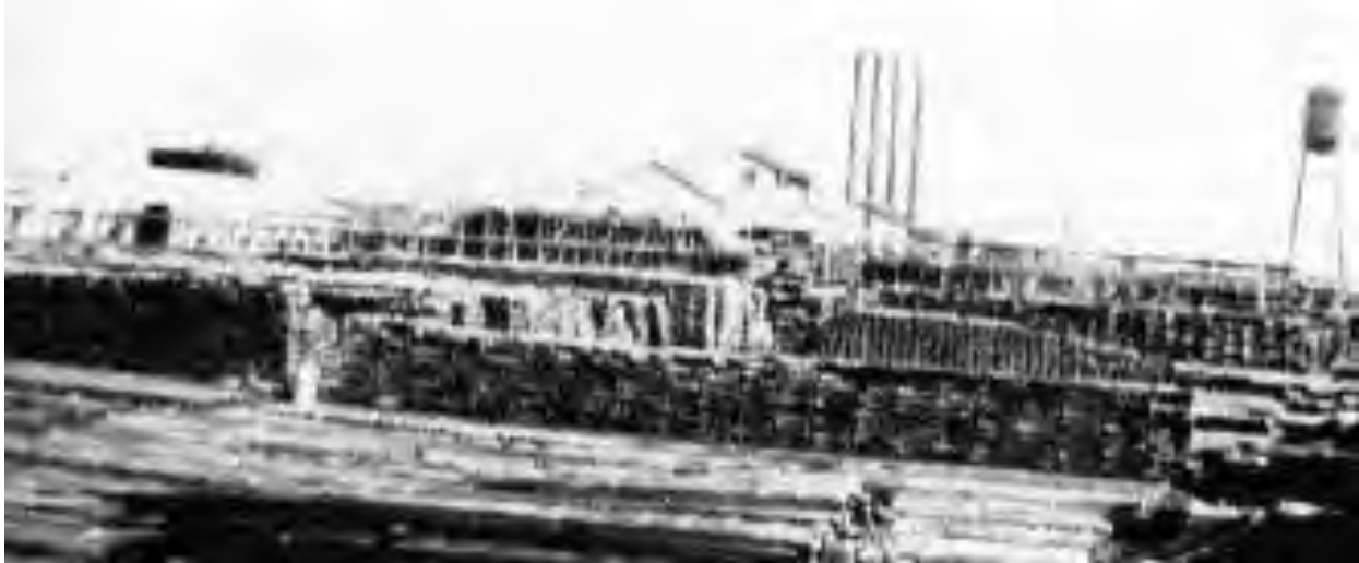
Figure 10: Union Cypress Company Lumber Mill (1916)
