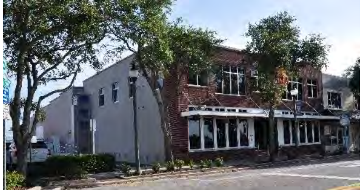
1002 E New Haven Ave
