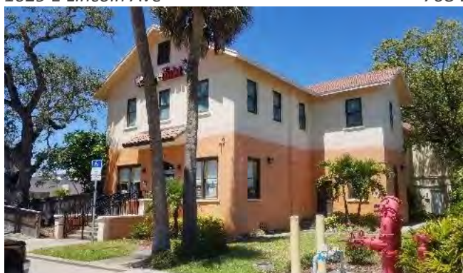
702 E New Haven Ave
