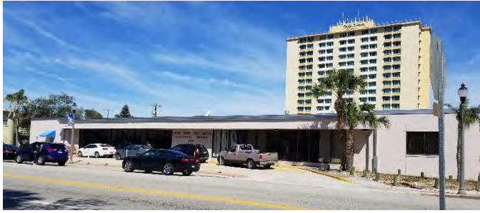
630 E New Haven Ave
