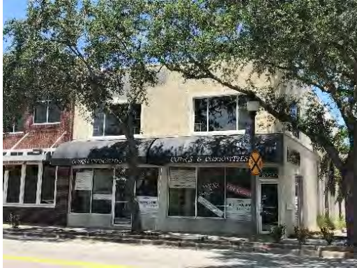
1010 E New Haven Ave
