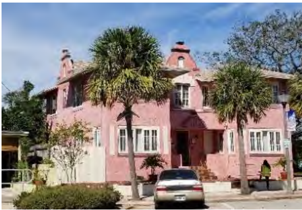
616 E New Haven Ave
