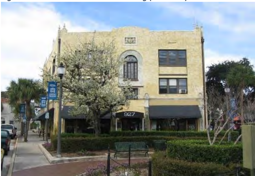
Figure 16: Melbourne Flat Iron Building (BR01410)
