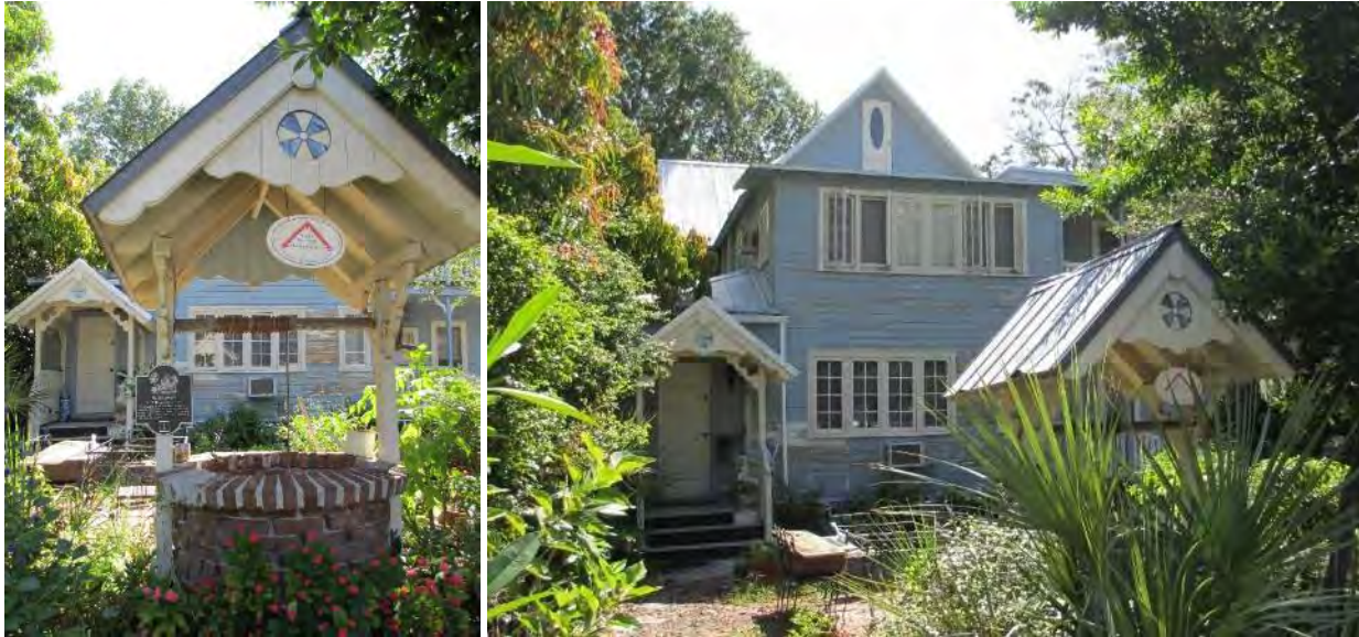
Figure 33: Eaton House (1809 Riverview Drive/BR01195)
