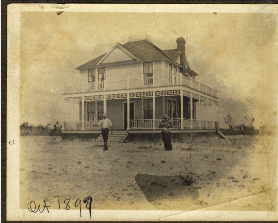
Figure 21: South Façade, 1897 and 2009
