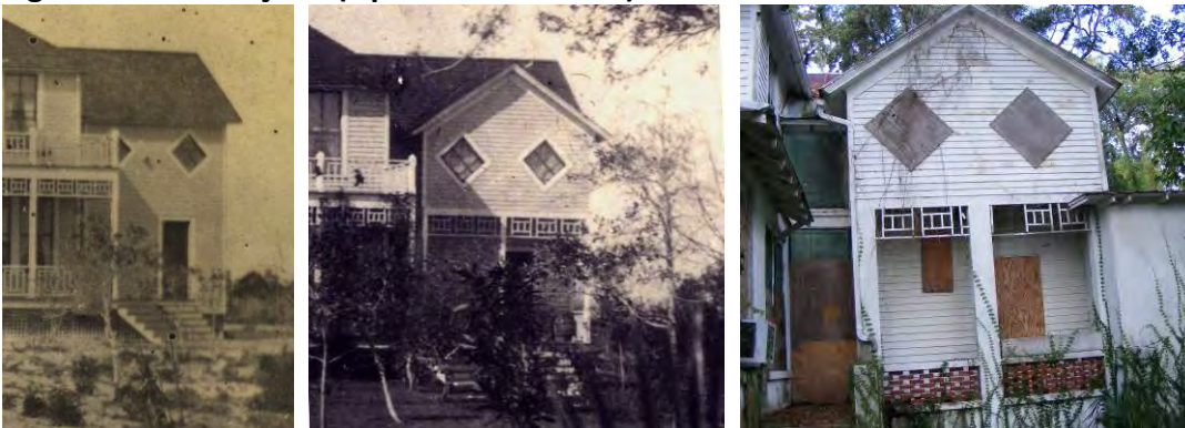
Figure 25: East Façade (Upstairs Bathroom)
