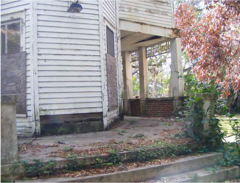
Figure 26: West Entrance to Masonry Porch
