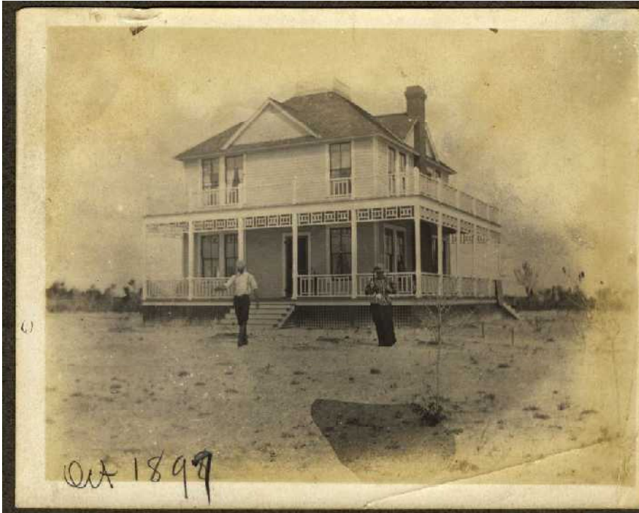
Figure 21: South Façade, 1897 and 2009
