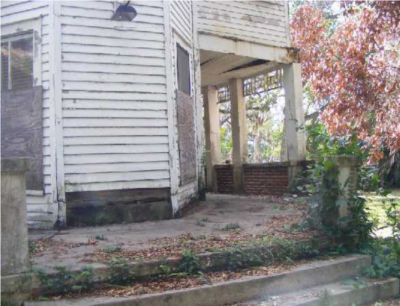
Figure 26: West Entrance to Masonry Porch
