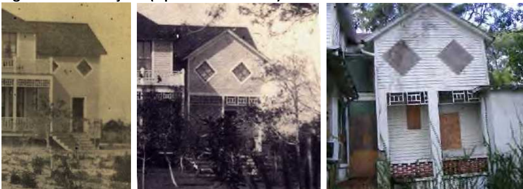
Figure 25: East Façade (Upstairs Bathroom)
