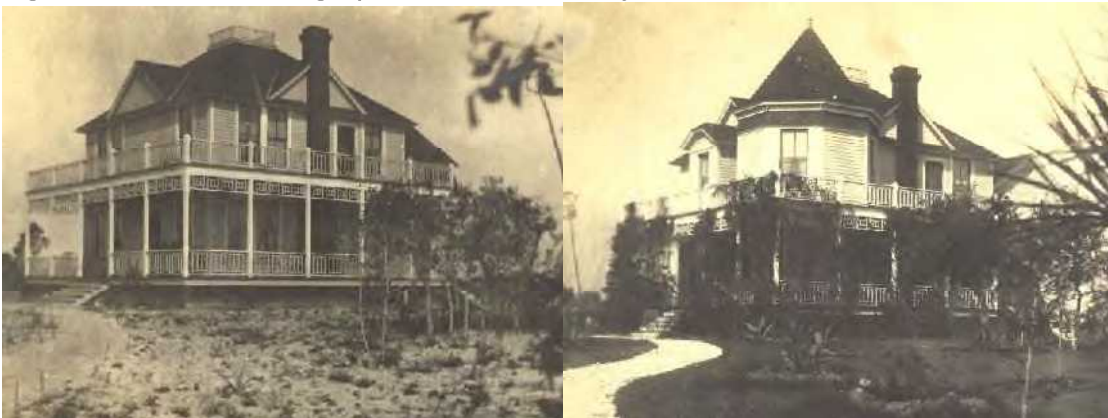
Figure 4: Historic Photographs – South/East Façades
